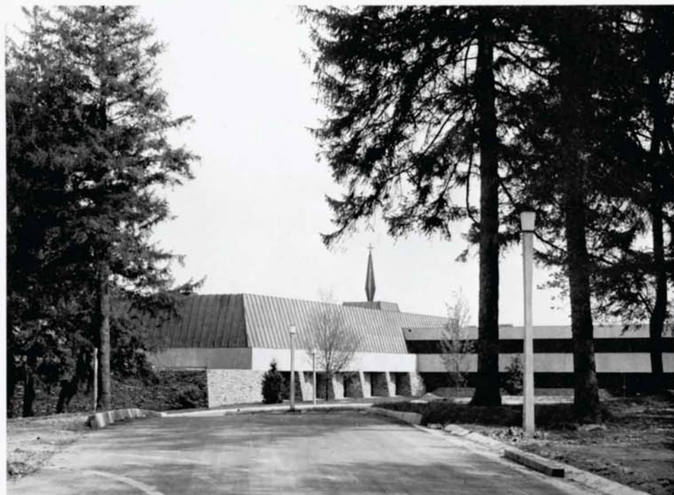
UPPER: Bon Secours Hospital, Baltimore (today) LOWER: Bon Secours Provincial House and Spiritual Center, Marriottsville, MD
